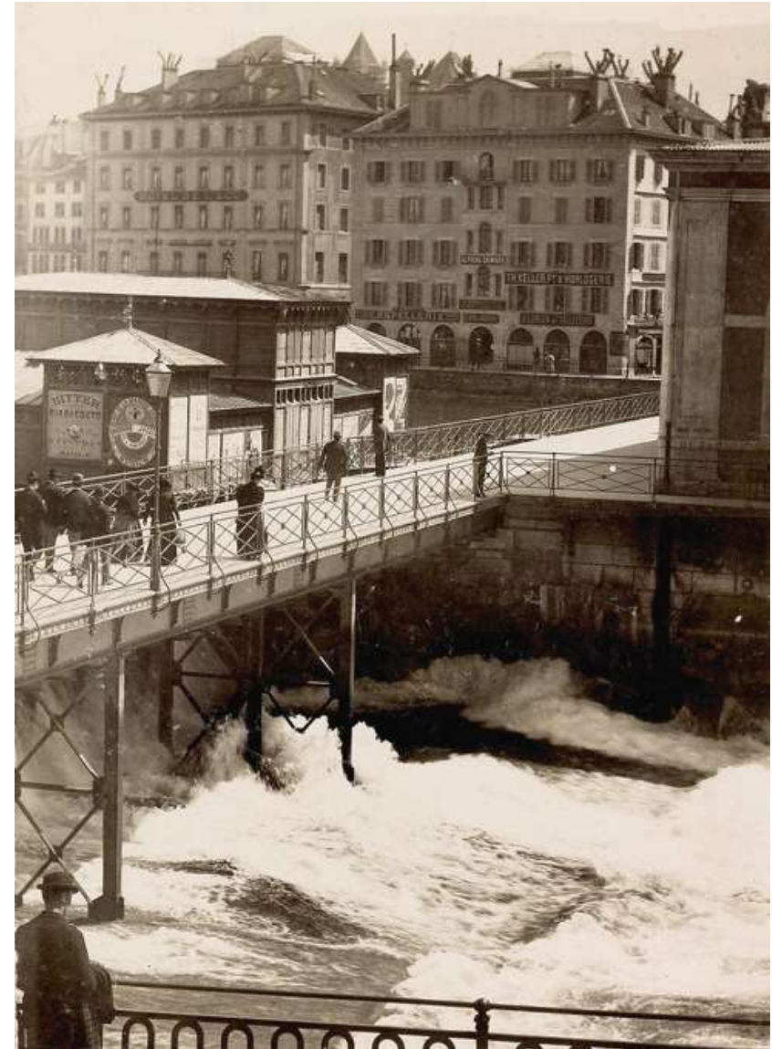
Figure d: the sluice gates of the Machine Bridge viewed from downstream of the bridge, between 1888 and 1898 (BGE, Genva Centre of iconography).
