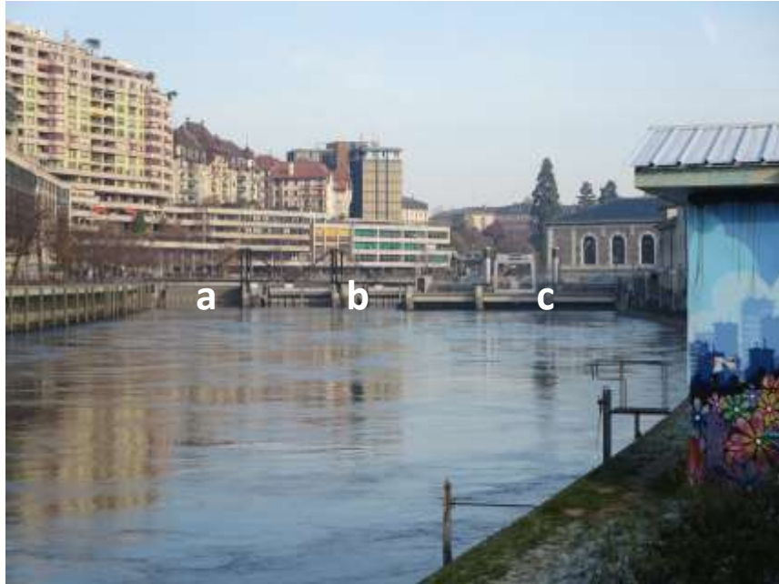
Figure c: dam and sluice of the Seujet, downstream view from the left bank of the Rhône River; a) sluice, b) gates regulating the river flow and Lake Geneva level, c) turbines.
