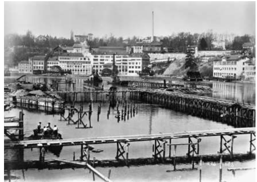
Figure 31: construction in 1885 of the Forces Motrices Building in Geneva. In the background, one can observe the hydraulic wheels which supplied energy to various industrial buildings in Saint-Jean: flour-mill, watchmaker and mechanical workshops. The hydraulic machines meant for providing drinking water to the city were moved from the «Pont de la Machine» to new buildings. The first «Jet d'eau» (water fountain) was meant to lower the pressure of unused water (BGE, Geneva Centre of iconography).
