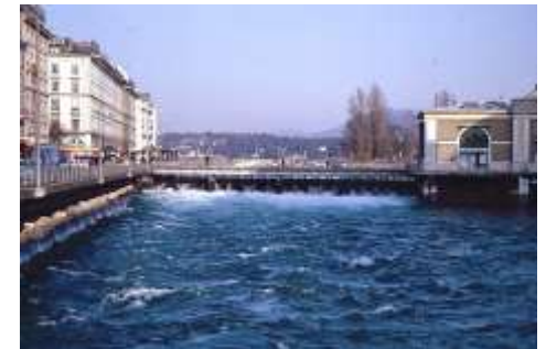
Figure b: the La Machine Bridge at the time when the Lake Geneva regulation was carried out through metal shutters underneath the bridge. This device, totalling 39 larch-wood shutters was constructed in 1887 (photo: view from the Belair Island, 1988).
