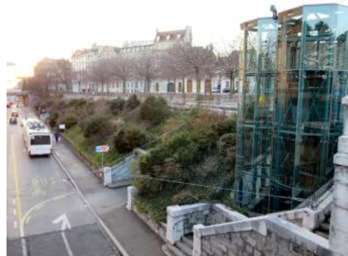
Figure b: Saint-Antoine Promenade and parking viewed from the bridge crossing the Boulevard Jaques Dalcroze. The construction of the parking has unearthed old fortifications of the town and the Saint-Antoine Delta.
