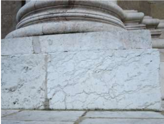
Figure c: base of a column at the cathedral entrance; white-coloured limestone referred to as « vermiculé » (see darker specks), with numerous stylolites (fine, zig-zag shaped dilution sutures).
