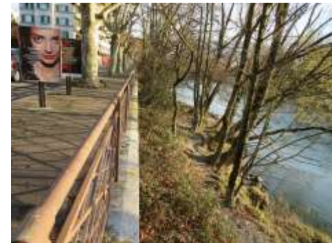
Figure b: upstream view of the Quai Ernest-Ansermet embankment, on the right bank of the Arve River. This man-made construction protects the areas of Plainpalais et La Jonction from centennial and millennial floods.
